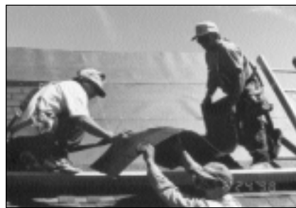
UNI-SOLAR solar shingle installation. Courtesy of United Solar Systems Corp.
